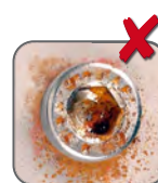
STAINLESS STEEL + NO STAINLESS STEEL = RUST
